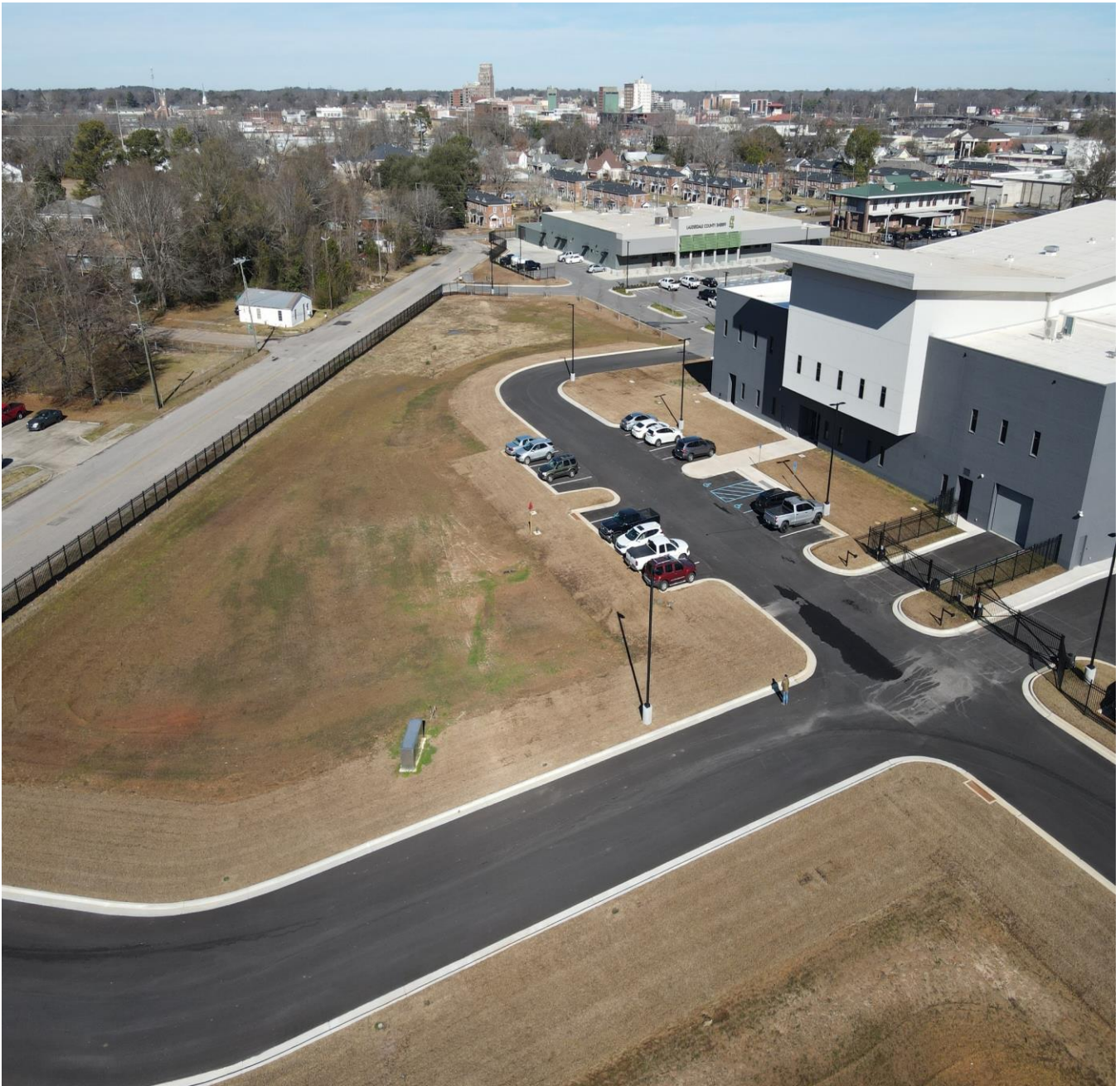
Overview of the back of the building Image 4. Considered as part of the Government Building & Entry Blvd Bid.
