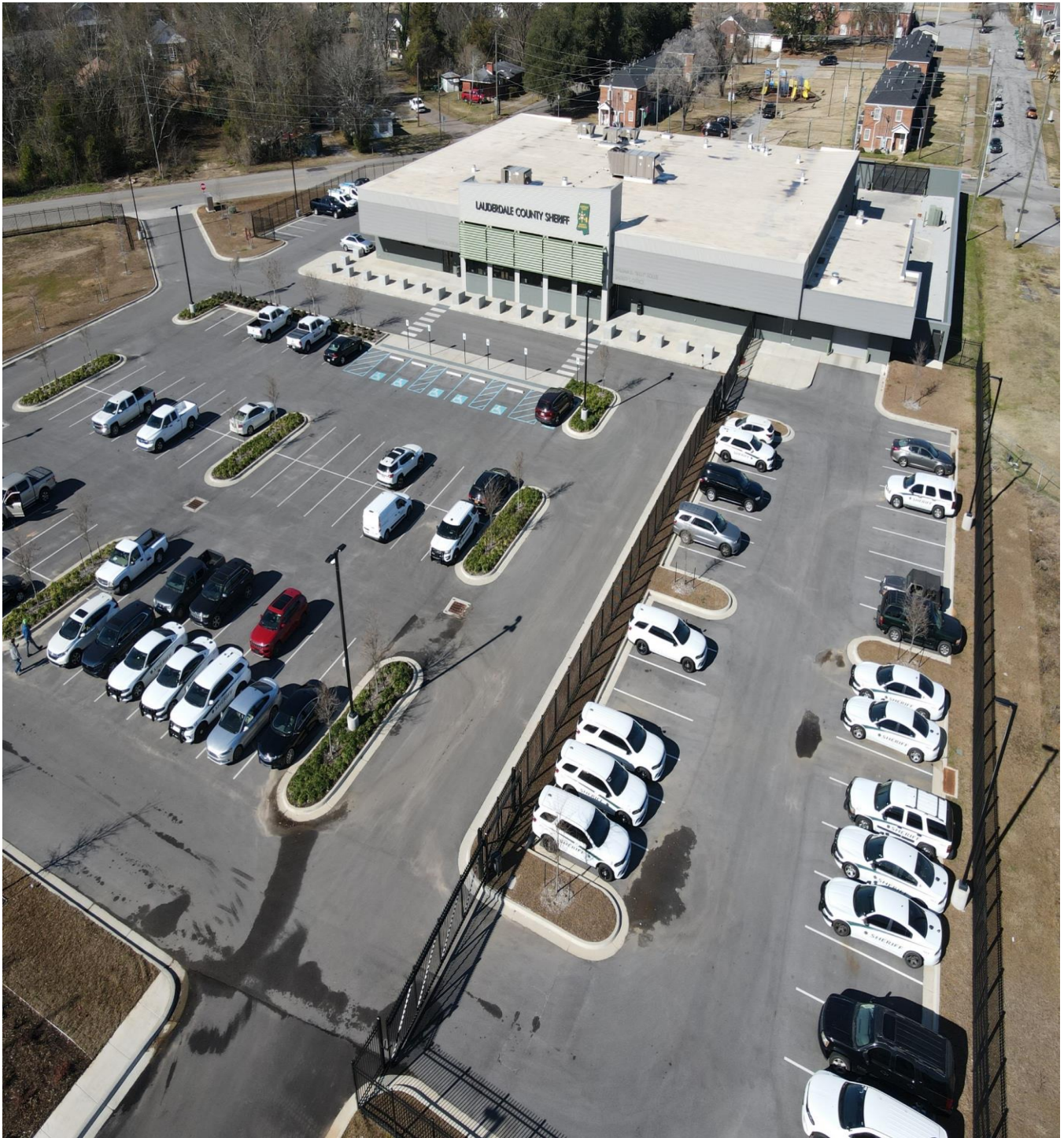
Overview of the Public Safety Building Image 1.
