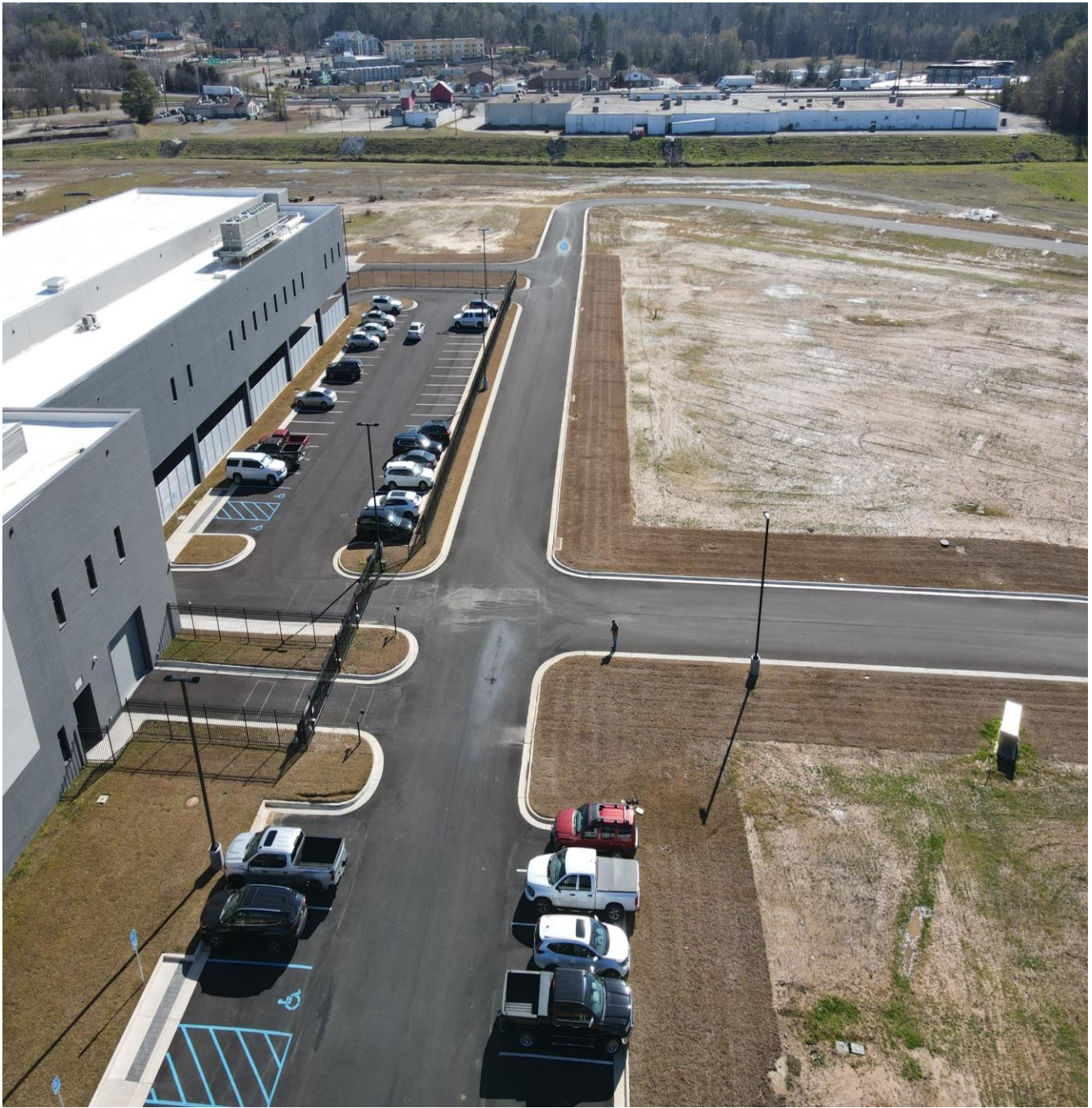
Overview of the back of the building Image 2. Considered as part of the Government Building & Entry Blvd Bid.
