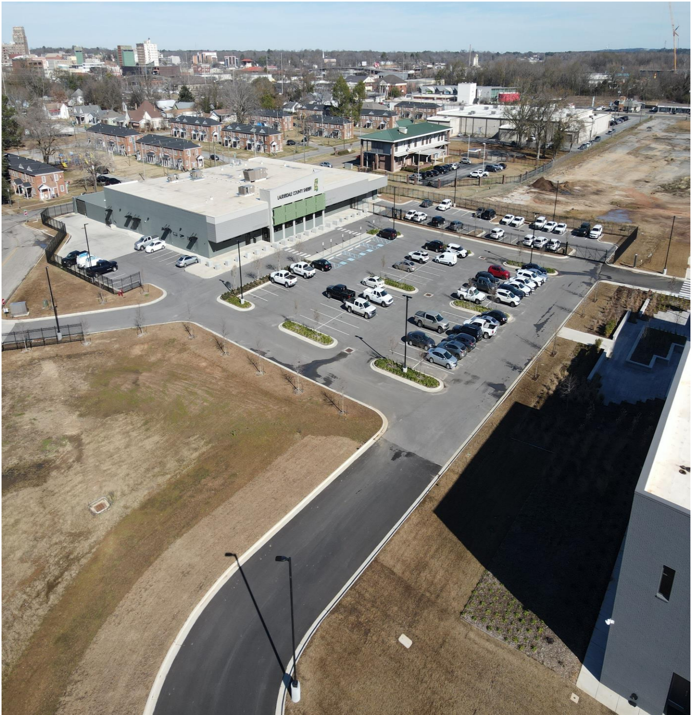
Overview of the Public Safety Building Image 2.
